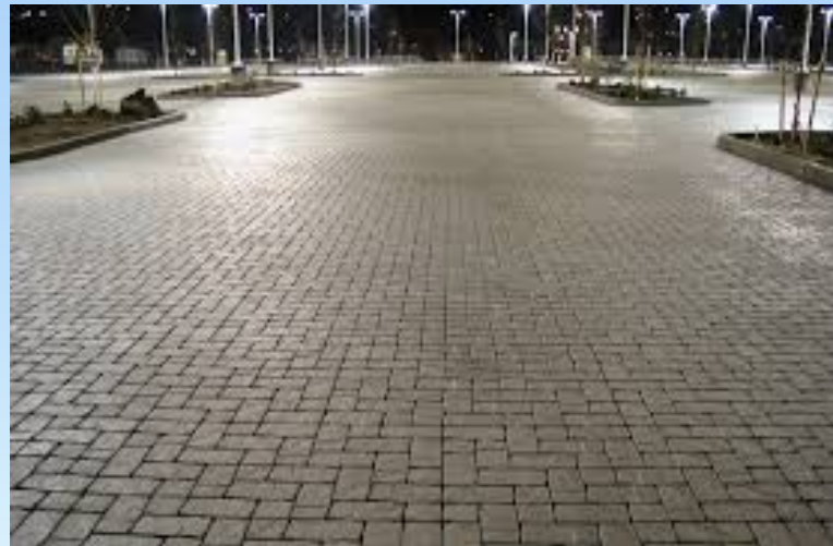
Image courtesy of advancedpavement.com
