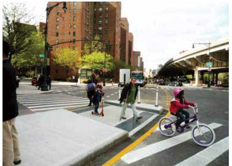
TOP: Sidewalks connect homes in the Mueller neighborhood in Austin, Texas. (Thomas McConnell Photography) ABOVE: In New York City, a variety of strategies—including signs, curb extensions, medians, and special markings—are used to keep pedestrians safe when crossing the street. (New York City Department of Transportation)
