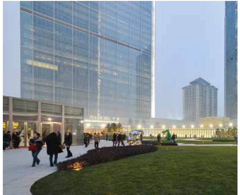
A green roof garden provides views of green space and access to nature at Chengdu International Finance Square in Chengdu, China. (Benoy Ltd.)
