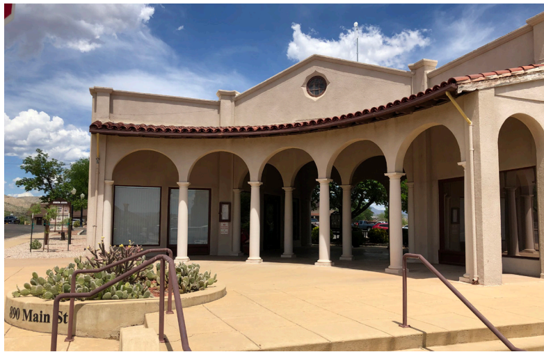
Figure 1 Town of Clarkdale Community Development Department Building
