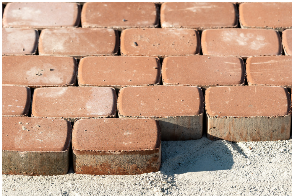
Figure 10 One example of permeable pavement includes bricks laid with a fine gravel underneath, which allows water to infiltrate the ground through the crevices between bricks
