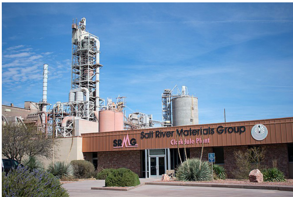
Figure 2 Phoenix Cement Company's Clarkdale plant, by Town of Clarkdale
