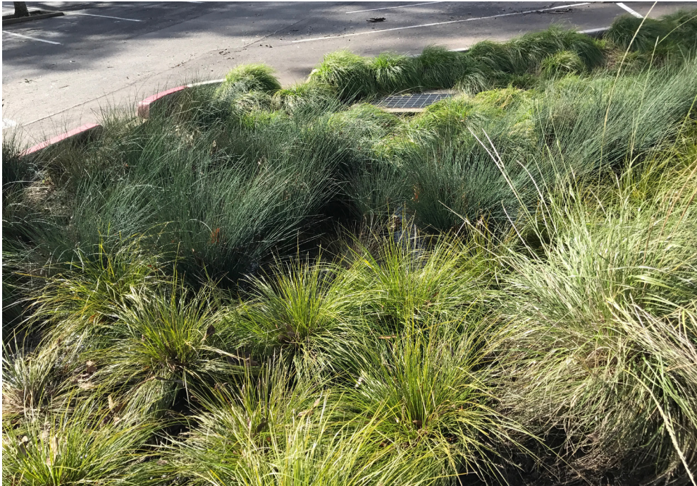
Figure 14 Bioswales are one LID tool that helps direct and collect stormwater runoff, allowing it to saturate the soil and replenish groundwater or sustain landscaping
