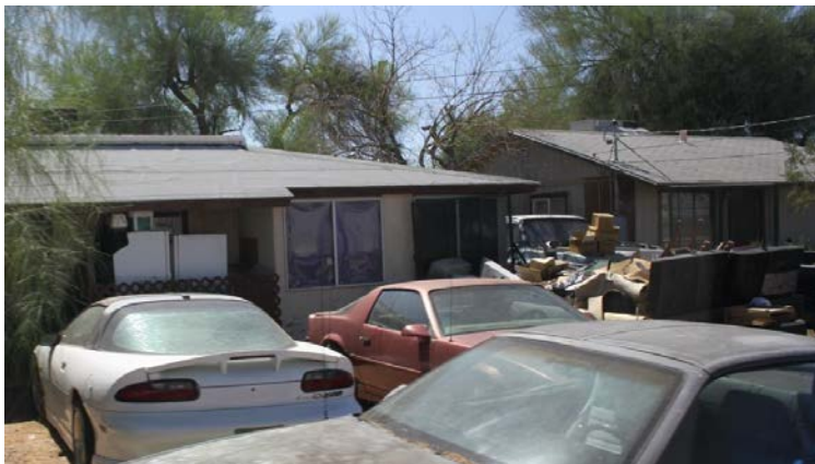
Figure 3. Combustible material stored next to a dwelling; source Gandhar Pandit
