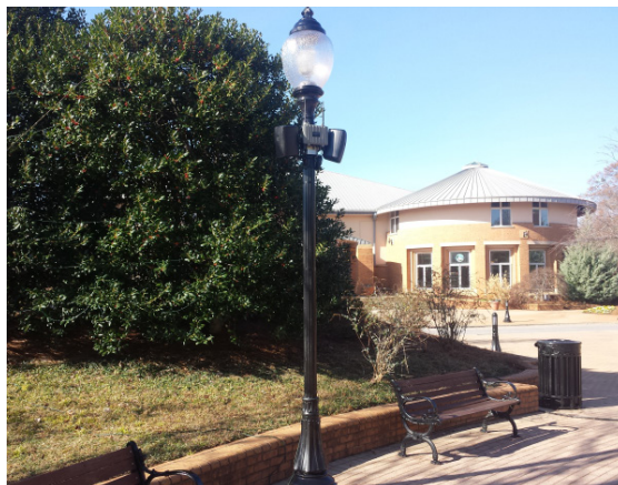
Figure 26 Example of StreetSounds hardware installed on a walkway lightpost
