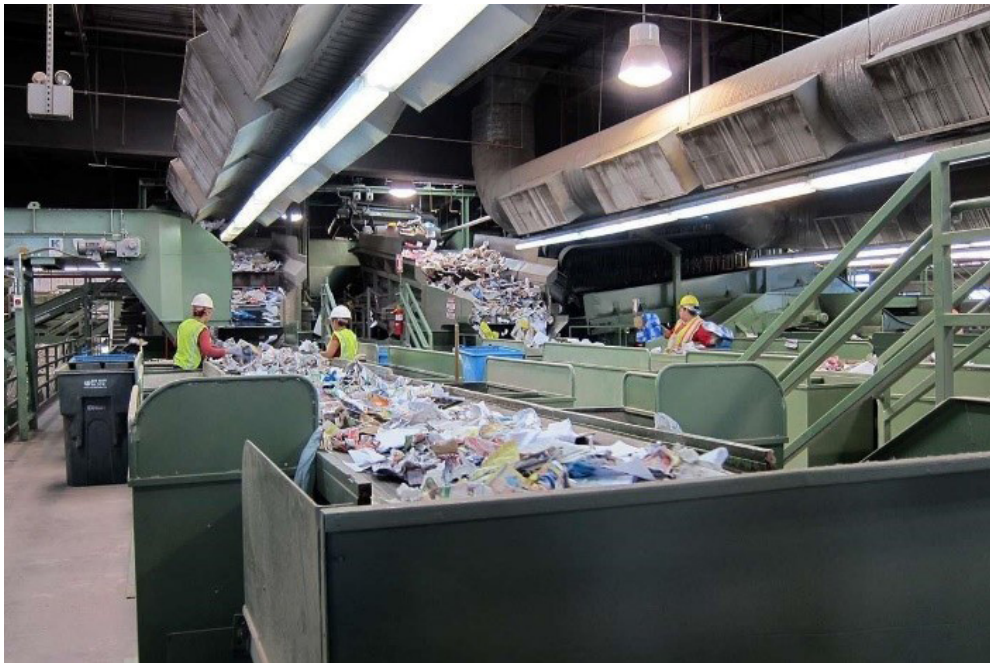
Figure 10 Phoenix North Gateway Transfer Station which includes an adjoining MRF.
