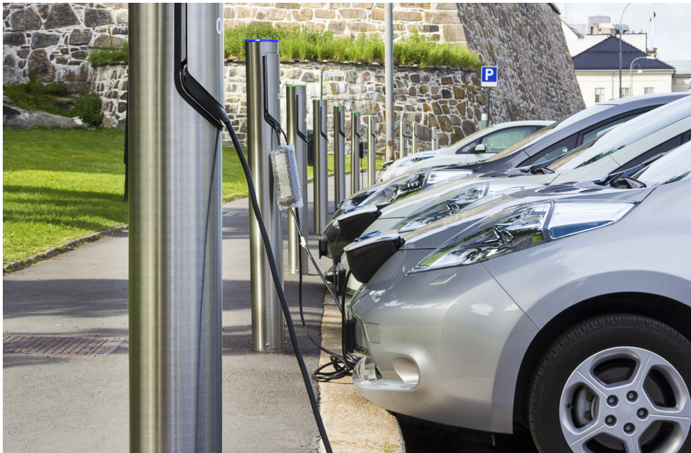
Figure 15 Strategically placed EV charging stations also convey a message to visitors, as a visual manifestation of the community's commitment to sustainability.
