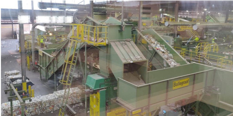
Figure 2 Sorting of recyclables at the Phoenix North Gateway Transfer Station
