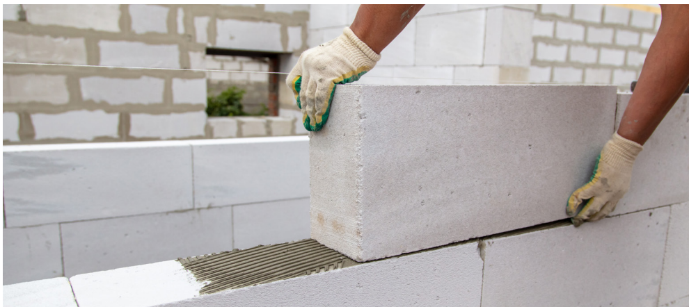
Figure 5 Laying foam concrete blocks for a residential foundation
