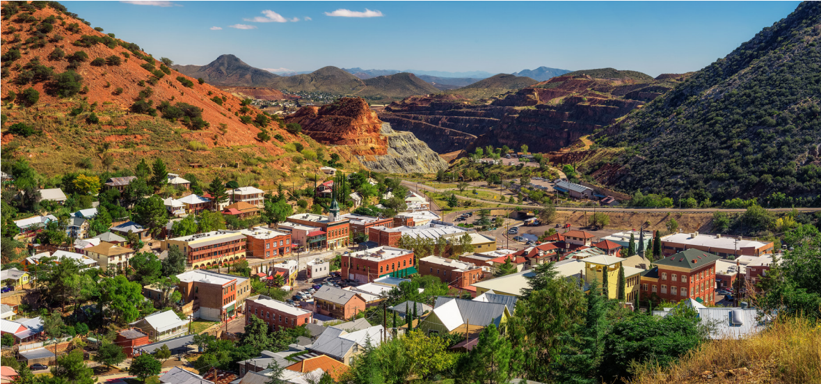
Figure 3 Aerial view of Bisbee's main downtown area
