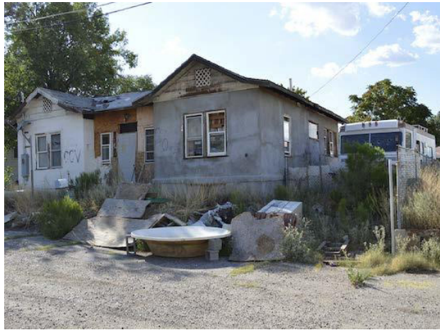
Figure 40 Example of a dilapidated residential property in Globe
